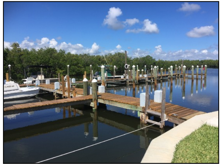
New Decking at the Marina
